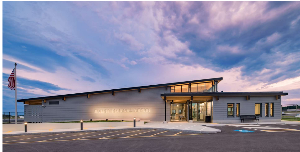
Figure 2-6: BVY Administration Building
